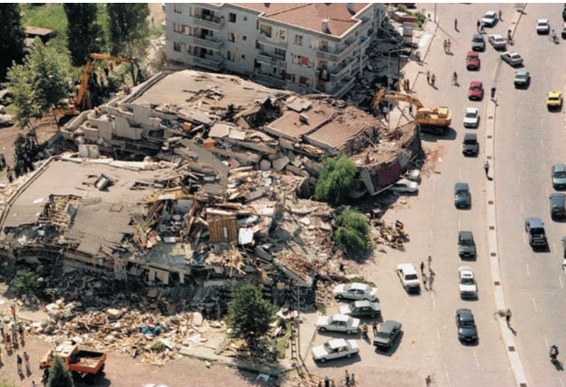
FIGURE P.3 Human-made cities cannot withstand the vibrations of a large earthquake. These apartment buildings collapsed during an earthquake in Turkey.
